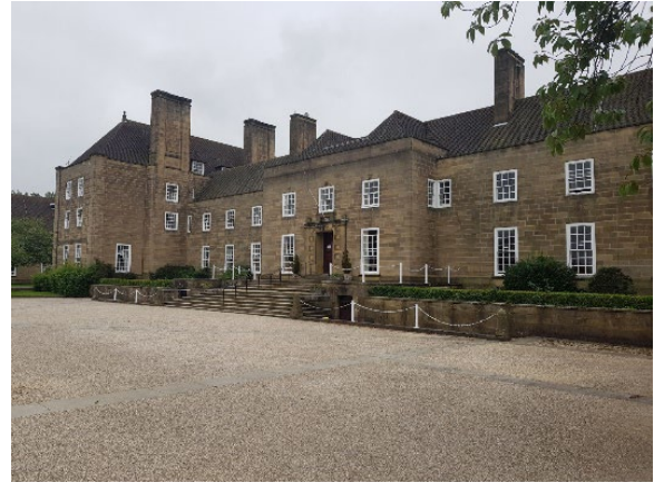
St. Mary's College, Durham City Asset type: College building and landscape
