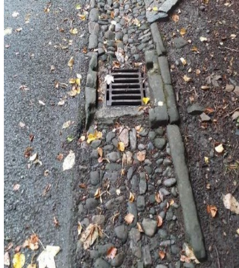
Cobbles and floorscape in Durham City Asset type: Floorscape
