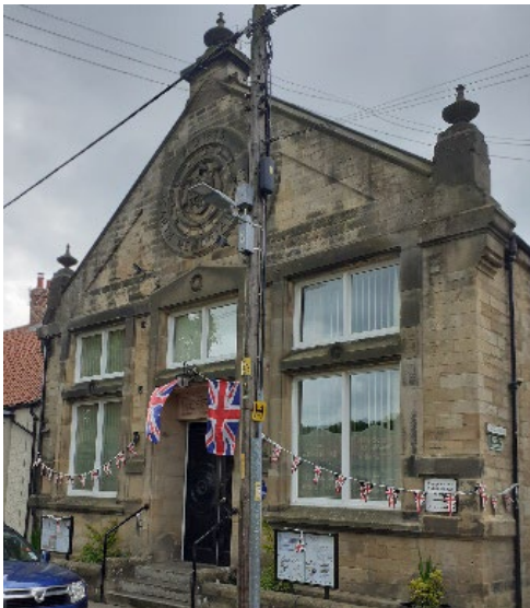
Scarth Hall, Staindrop Asset type: Building
