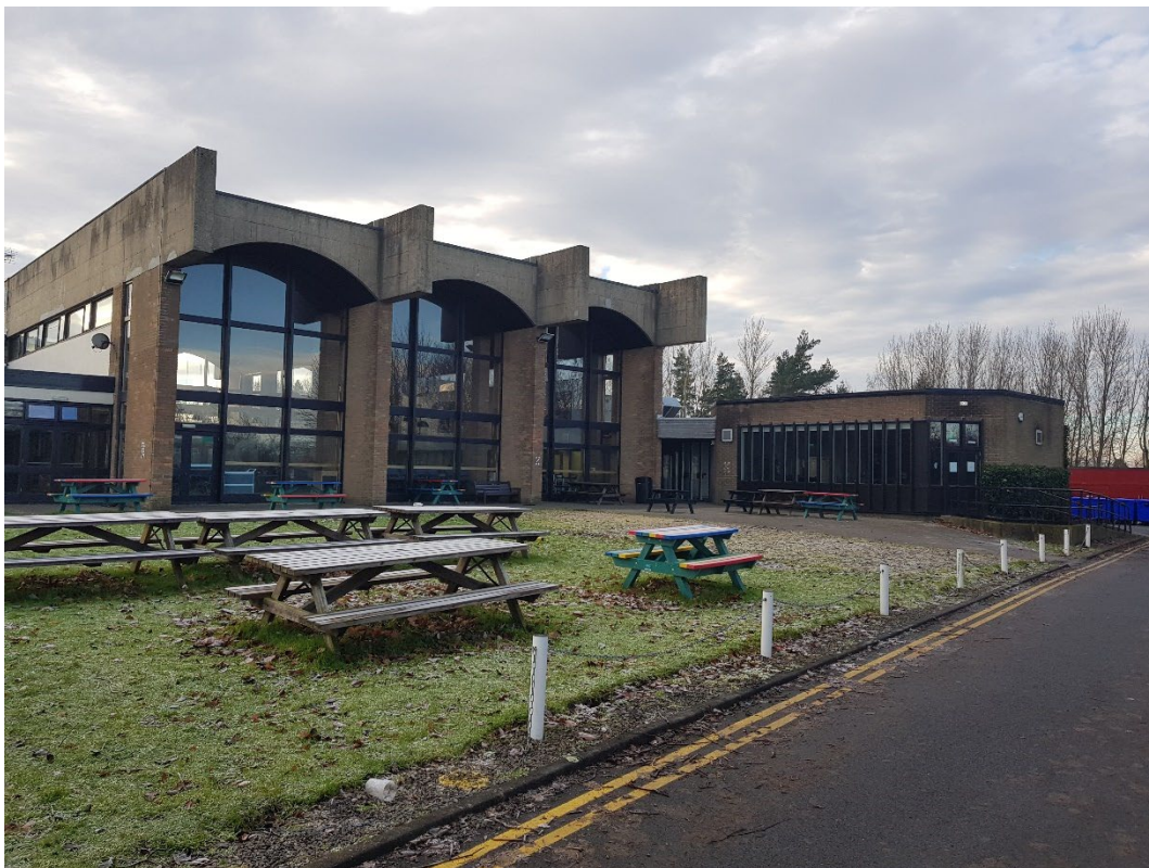
St. Aidan's College, Durham City. An asset identified on the Durham City local list.
